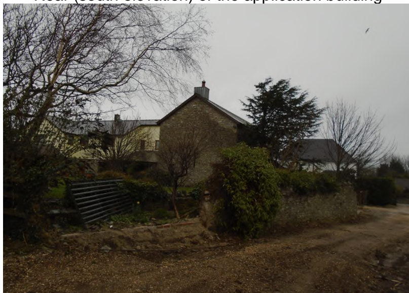
Rear (south elevation) of the application building
